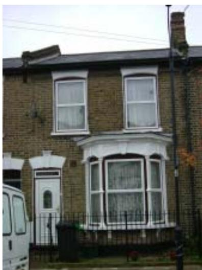
Replacement windows in upvc are different in appearance to the characteristic timber framed sliding sash windows seen across the conservation area. The door is also of non-traditional design and materials and is set further forward than other doors.
