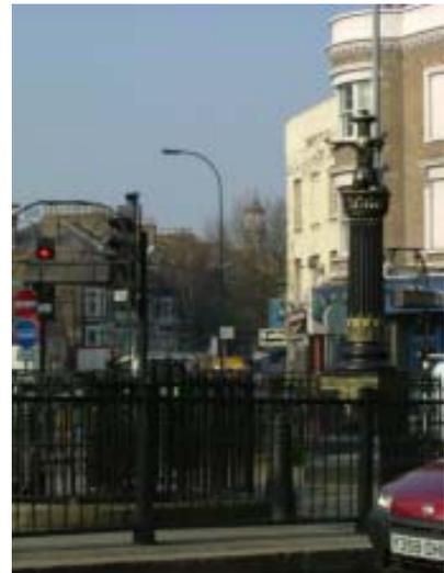
This cast iron column was modelled on an Egyptian designs by Alexander 'the Greek' Thomson. The column vented the public conveniences beneath and was installed in 1897. It is grade II listed.
