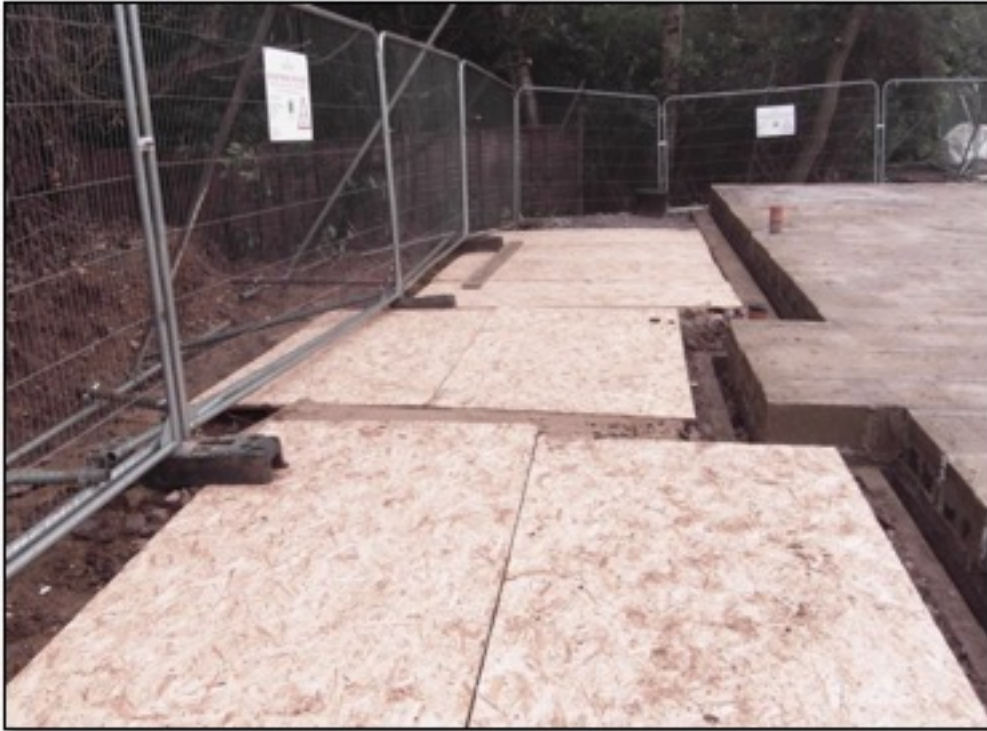
Fig.1 Heavy-duty OSB boarding over a depth (min. 50mm) of sharp sand and/or wood chip between the tree protection fencing and the foundation line of new development. An effective way to protect roots, which grow in the soil beyond the position of the fencing.
