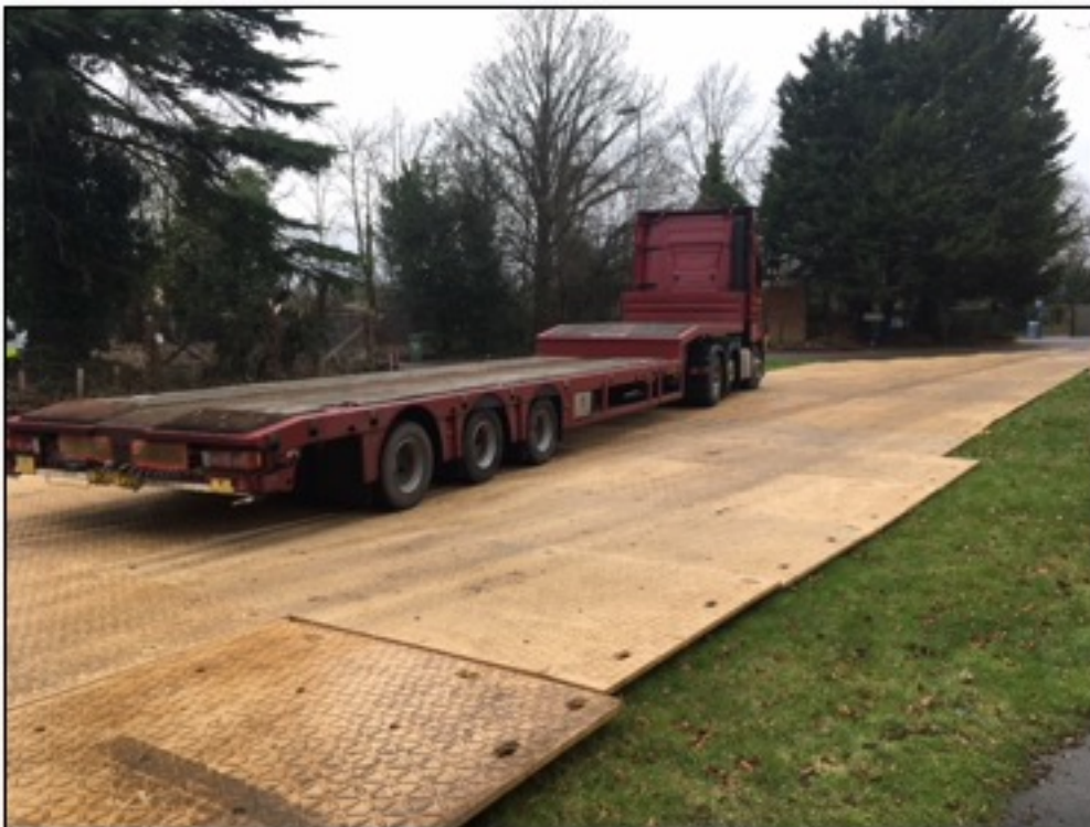
Fig.2 Heavy-duty metal ground plates laid on minimum 75mm depth sharp sand/ woodchip, fixed in position with road pins.
