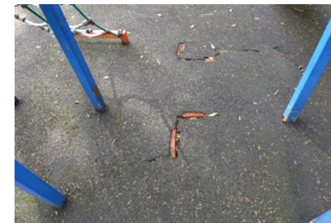
Bound rubber crumb surface failing
