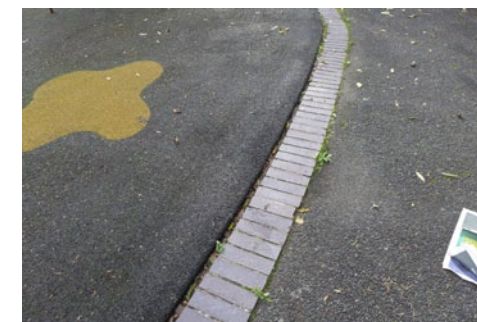
Bound rubber crumb surface failing
